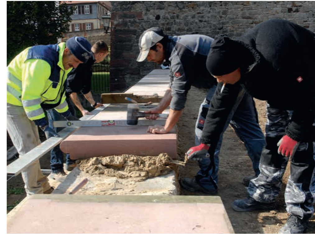
The masonry team completing the wall with the cover plates
