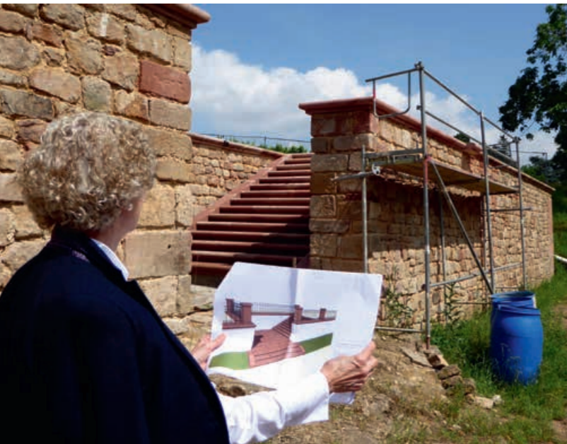
Construction of the lowest retaining wall
