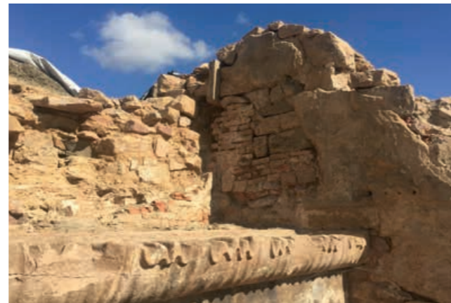
Numerous toothings on the overflow basins ensured a refined overflow of water
